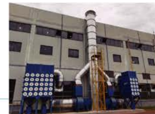
•SG Zhejiang dust removal equipment installation project
